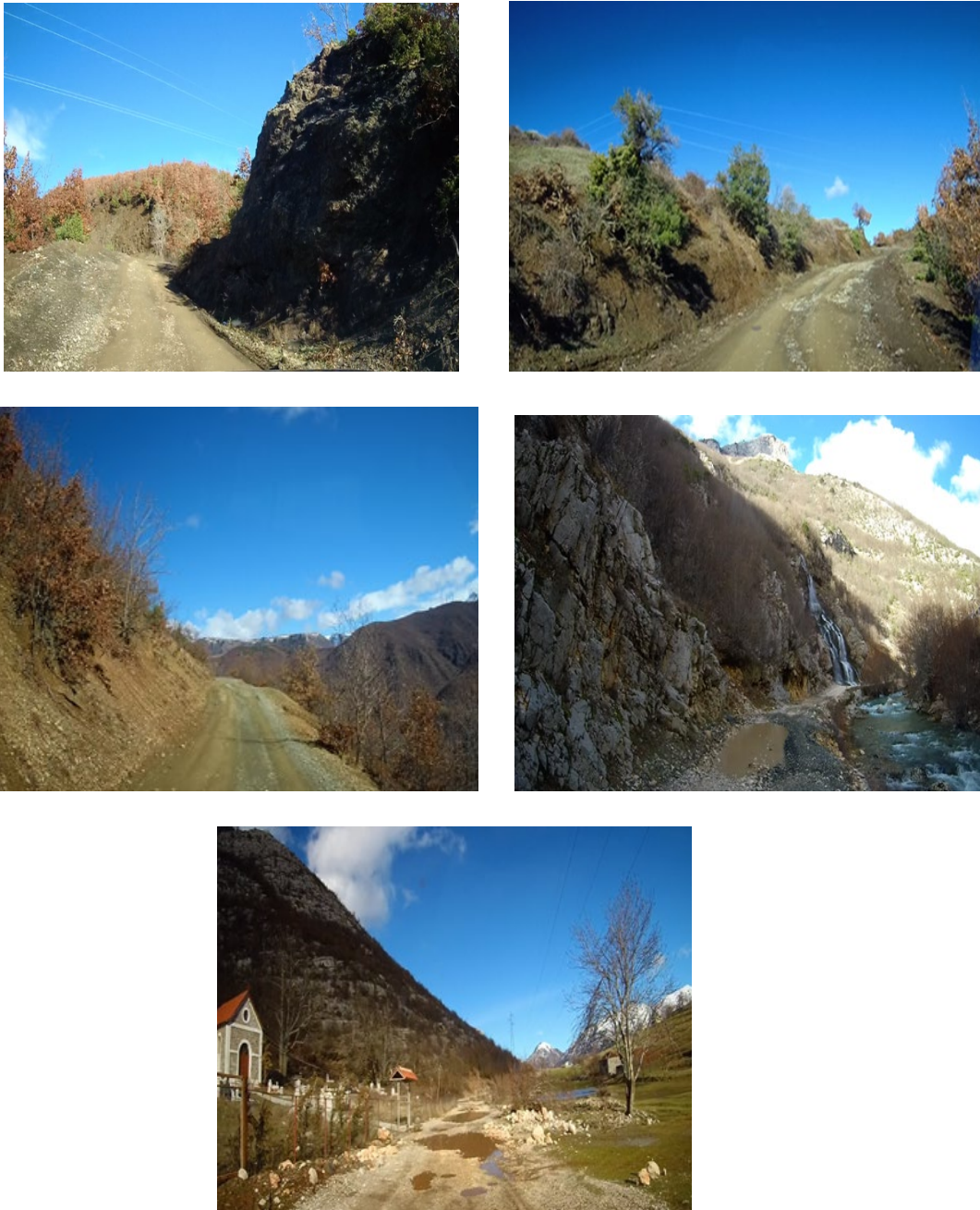
Figure 3: Existing condition of the road
